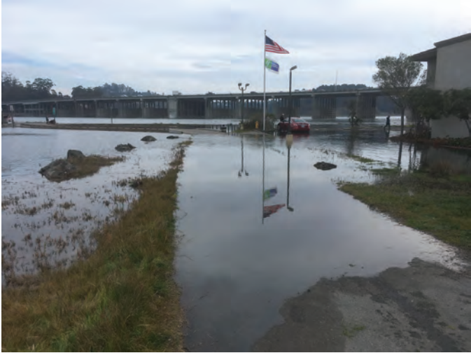
EDGE WEAR AT AREAS WITH KING TIDES
