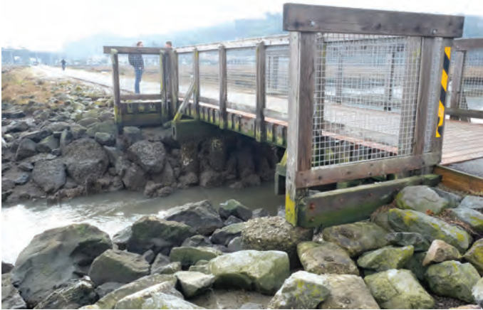
BRIDGE 2 - SOUTH BOTHIN MARSH CHANNEL
