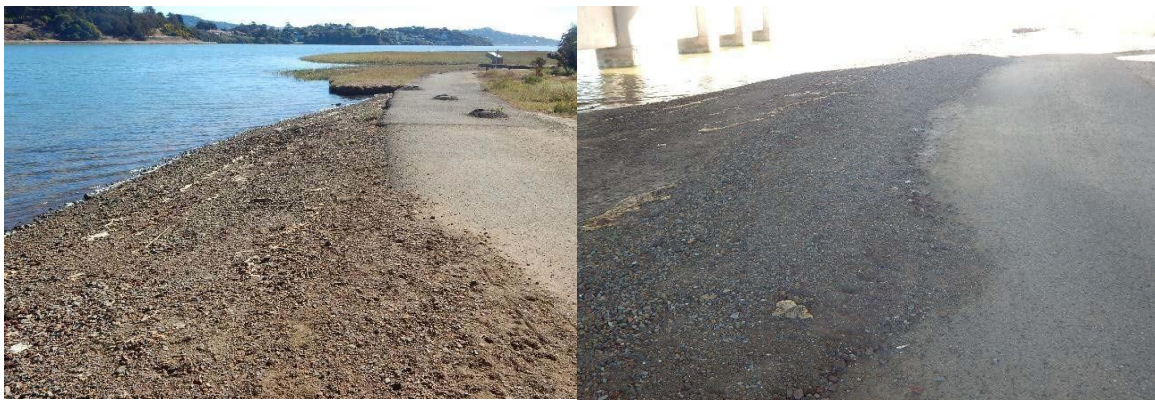
Figure 1.14. Gravel and sand berm accretion by wind-waves in Richardson Bay under the 101 Highway, south of Bothin Marsh. Local shoreline erosion of fill supplies the coarse sediment. Waves deposit a swash bar over the edge of the paved path. September 2017.
