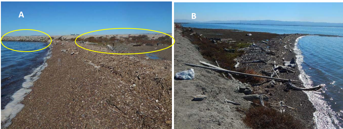
Figure 1.13. Gravel bay barrier beach formed from erosion of historic landing fill is shown at Newark salt ponds west of Coyote Hills, San Francisco Bay. (A) Unvegetated levee exposed to waves is armored with concrete slabs and rubble. (B) Salt pond levee in lee of barrier beach supports salt marsh and a vegetated levee slope. October 2014
