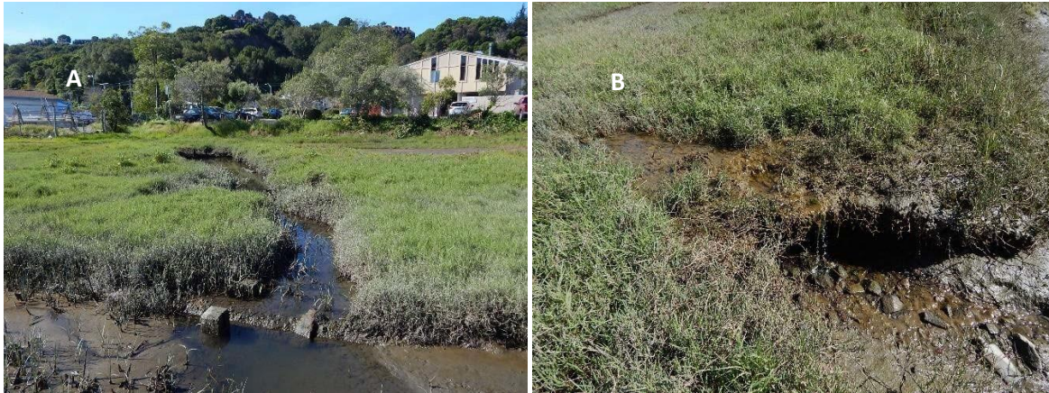
Figure 1.35. Old artificial fill and buried structures restrict eco-geomorphic development at South Bothin Marsh. (A) A buried pipeline exposed at the bed of a ditch acts as a grade control structure, preventing the ditch from achieving its equilibrium depth with its upstream tidal prism. (B) Resistant angular gravel in artificial fill along the north bank of Coyote Creek inhibits rapid channel incision and tidal creek evolution through the salt marsh surface (also see Figure 1.34 above). April 2017.
