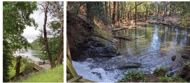
Wooden deck at the top of the spillway at Lake Lagunitas (left), bottom of the spillway next to picnic area (right)
